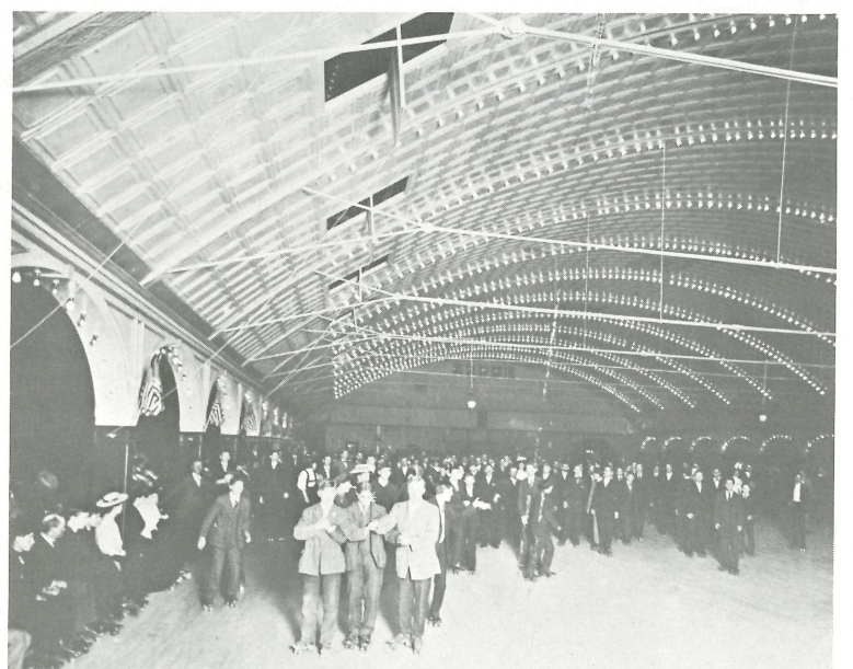
Barrel vaulting and skylight windows for ventilation characterize this unidentified arena in San Francisco, Calif., 1907. (Gift of Ernie St. Germain)
