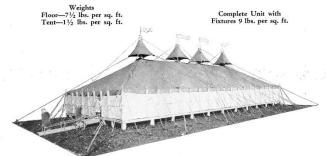
The tents used poles with steel joints and four foot hardened steel stakes. The finest un-oiled Manila rope stood alongside galvanized steel cables, unaffected by weather. Wall curtains rolled up to allowed plenty of light and fresh air. With skate and clothes racks, rails, and all fixtures, this complete unit quickly set up and knocked down without the use of a nail.
